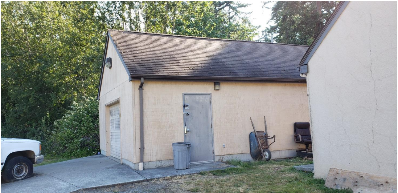
New Garage Exterior
