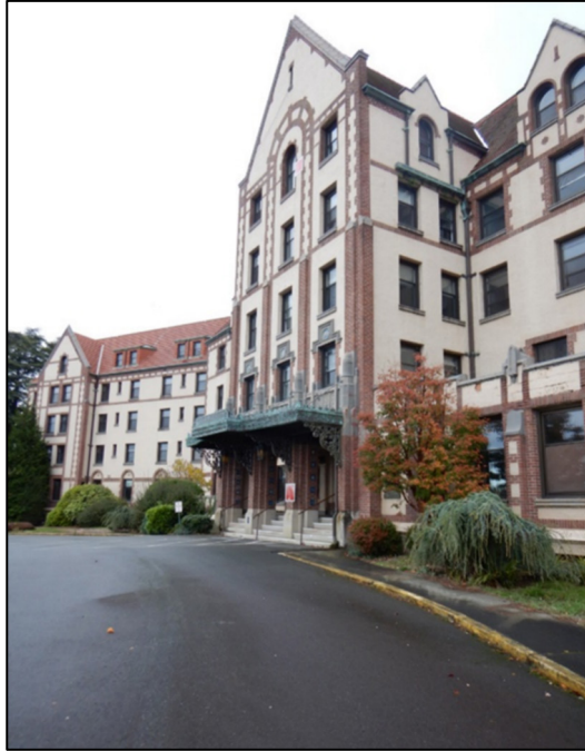
Photo ADA9 Passenger Loading Zone at the Main Entrance
