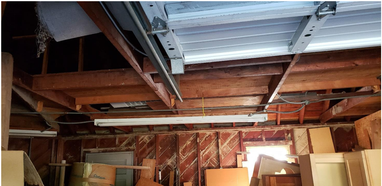
Old Garage Interior
