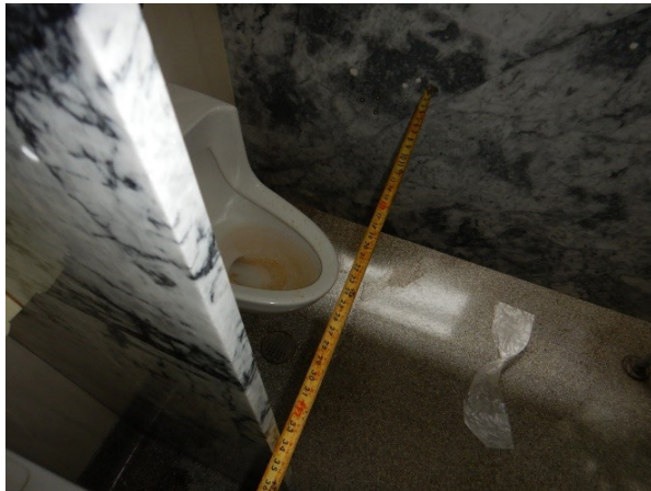
Photo ADA20 Front Approach
