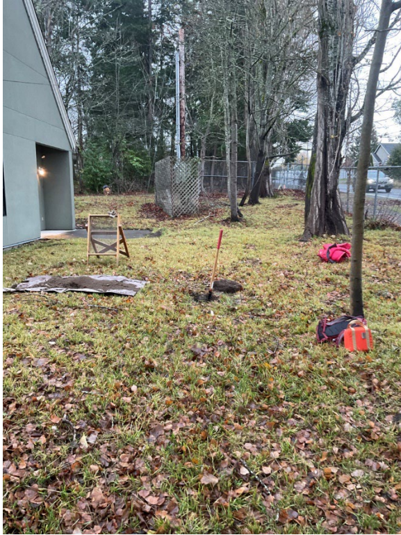
Figure 6-18. Overview SP-24 (view to east).
