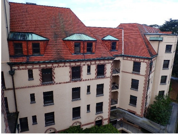
Photo BE1 Typical Roof
