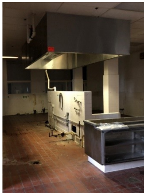
Photo M13 Decommissioned Commercial Kitchen
