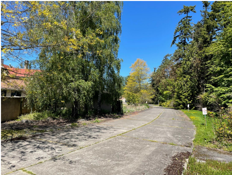
Figure 6-4. Overview of proposed demolition area on the driveway/road SE of the main building (view northeast).
