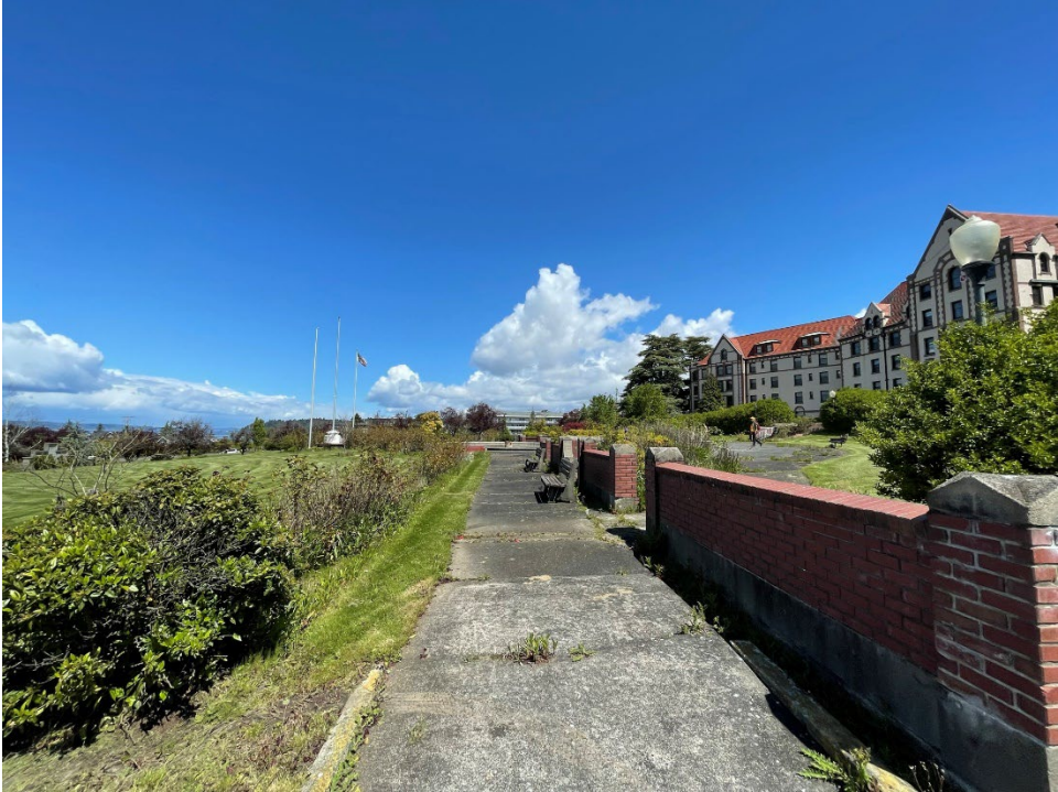
Figure 6-1. Overview of proposed demolition area on the east side of the property in front of the main building (view north).
