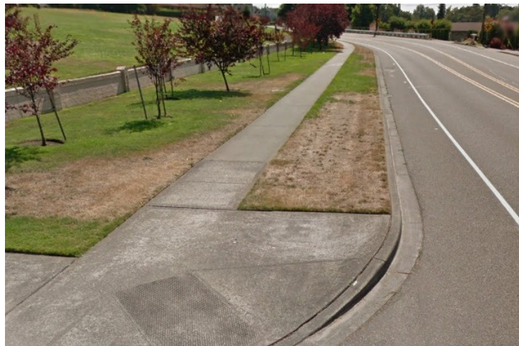
Photo C1 Marine View Drive Typical Frontage Section
