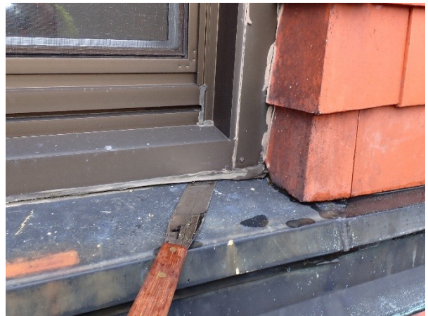
Photo BE6 Typical Window Seal
