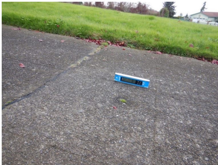
Photo ADA2 Slope of Walking Surface (Street to Parking)
