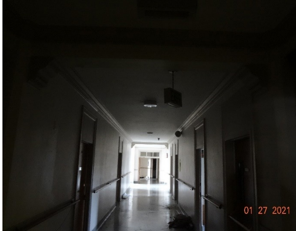
Photo E15 Surface mounted lighting fixture in corridor
