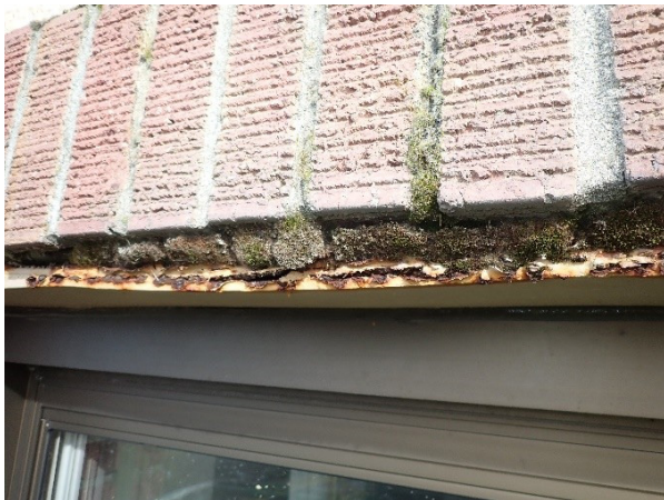
Photo BE5 Typical Lintel Supporting Brick
