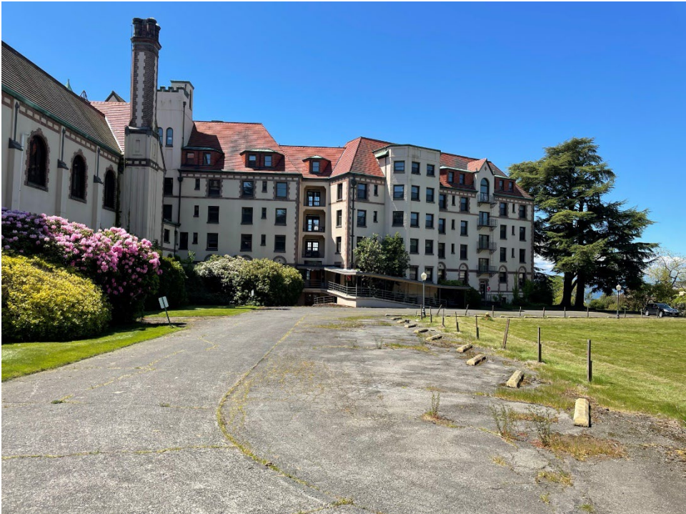
Figure 6-2. Overview of proposed demolition area on the north side of the building (view west).
