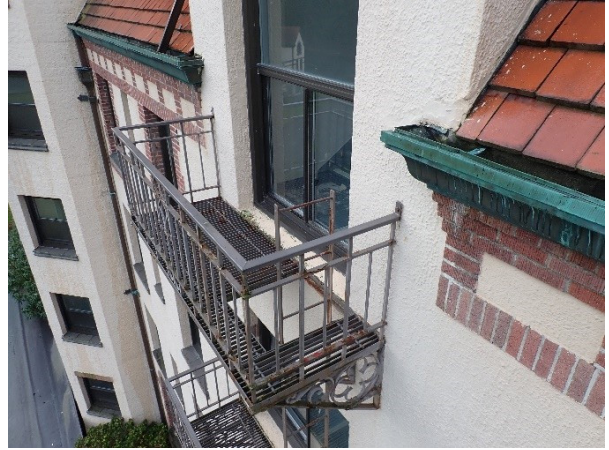
Photo BE2 Typical Wall & Fire Escape
