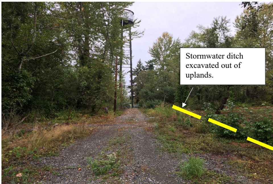
Photo 2: Looking north at a ditch excavated to convey run-off. August 31, 2023.
