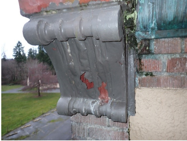
Photo BE7 Typical Ornamental Terra Cotta
