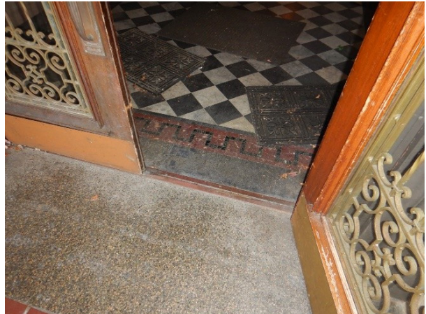
Photo ADA13 Main Entry Threshold
