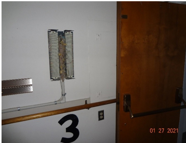
Photo E17 Corridor receptacles in fair condition
