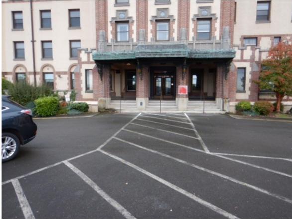
Photo ADA4 Accessibility Route as Viewed from Accessible Parking
