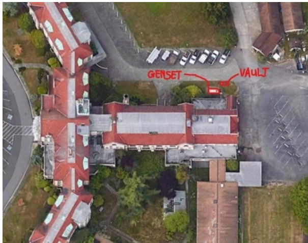
Photo E1 Aerial view utility/generator location
