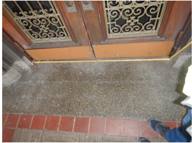
Photo ADA11 Main Entry Door Widths, >32 inches
