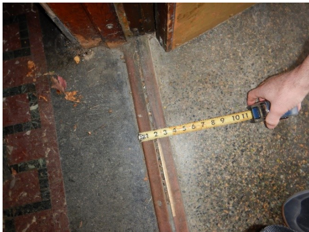
Photo ADA14 Main Entry Threshold Width
