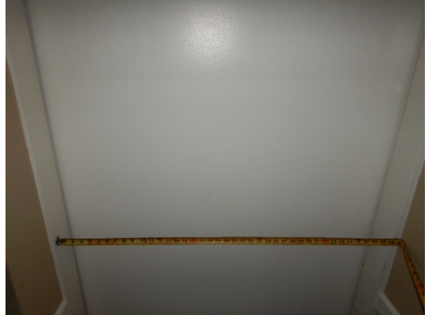
Photo ADA23 Elevator Clear Width
