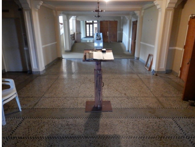
Photo ADA24 Ramp to Back of House
