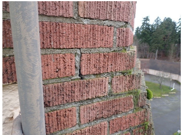
Photo BE4 Typical Wall Brick
